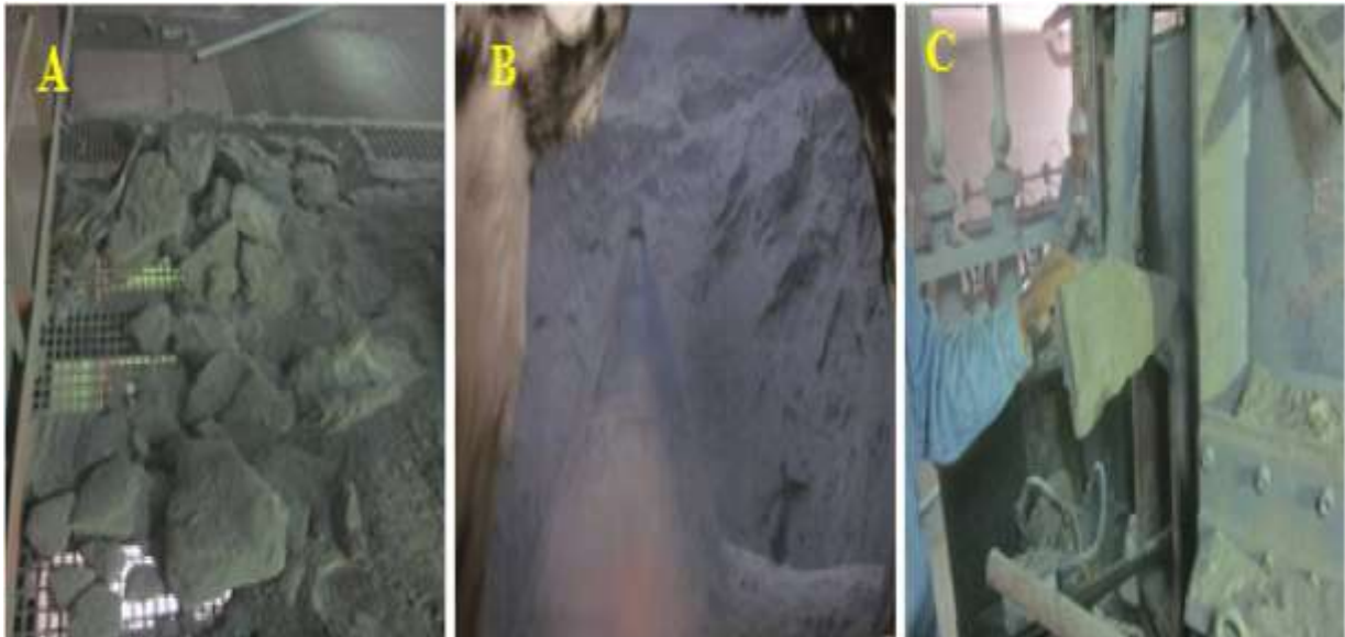
Fig. 6. lump formation inside cement silos.
